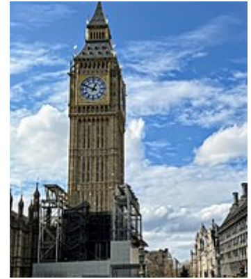
Elizabeth Tower with the scaffolding mostly removed, March 2022
