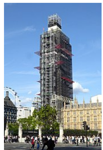
Scaffolding erected in 2017 to allow worker access
